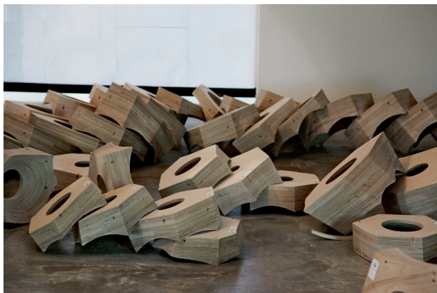
Fig. 10: Various unique voussoirs that compose the vault.
